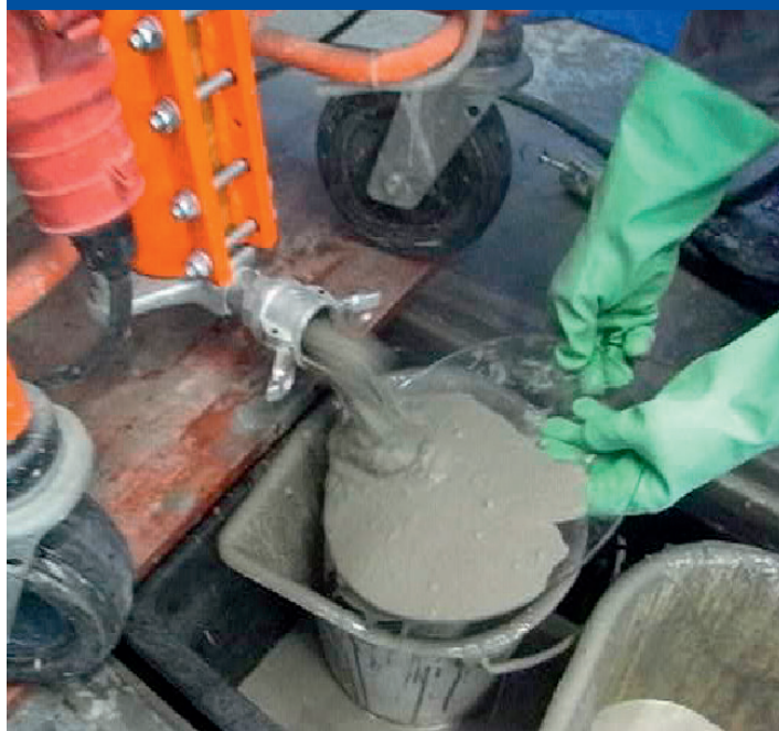
Field tests with screw mixing pump
